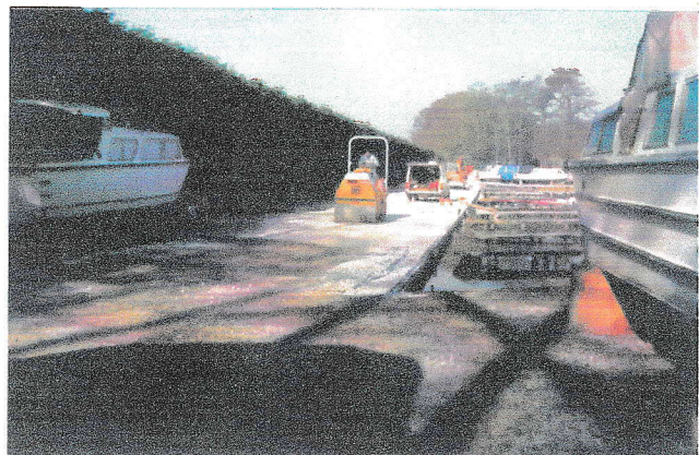
Repiling 'Dorfold Basin' and installing new stagings, circa 1998
